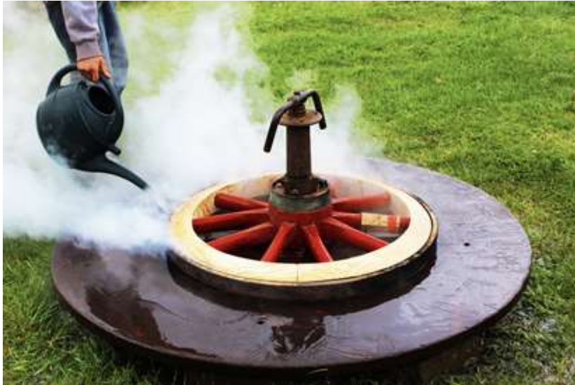
Rapid cooling the new tyre onto the wheel
