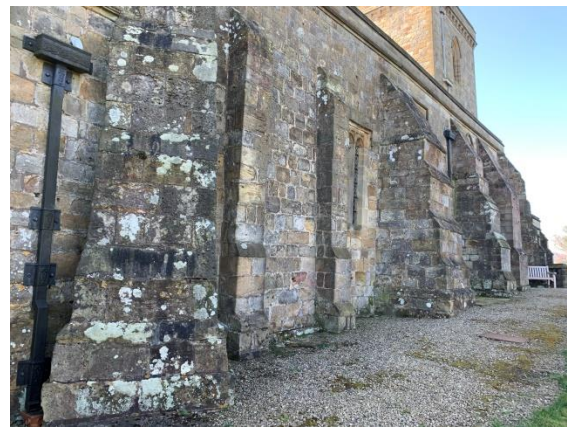
Buttresses supporting the north wall
